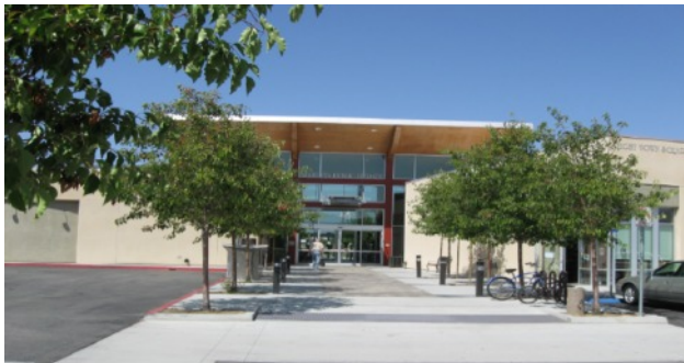
The Murrieta Public Library
